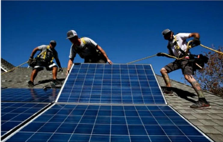
Vivint Solar workers install rooftop solar panels. Anne Cusack/Los Angeles Times via Getty Images
